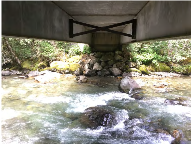
Right Bank Abutment when facing downstream
