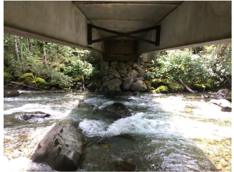
Left Bank Abutment when facing downstream
